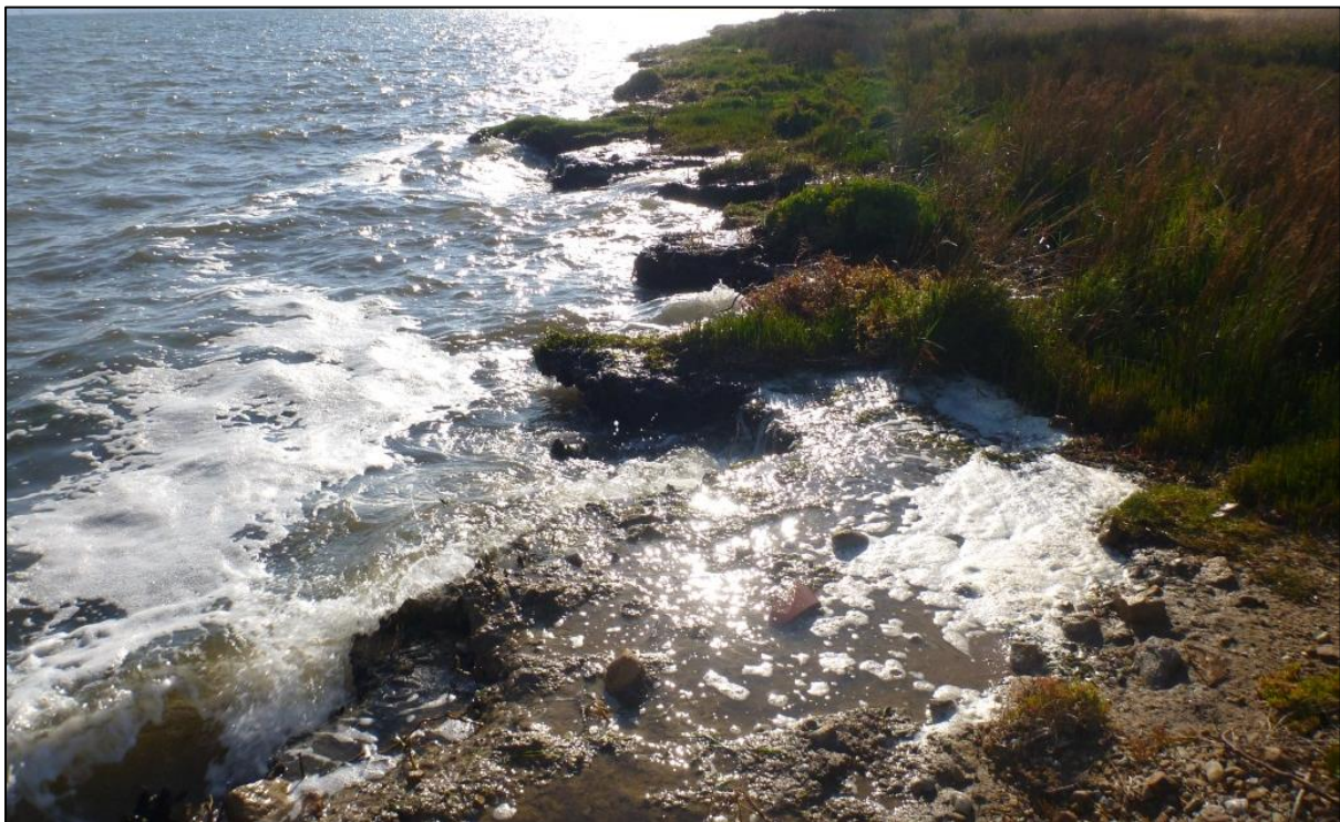
Figure 4-2 Erosive Section of Shoreline between Paynesville and Eagle Point
