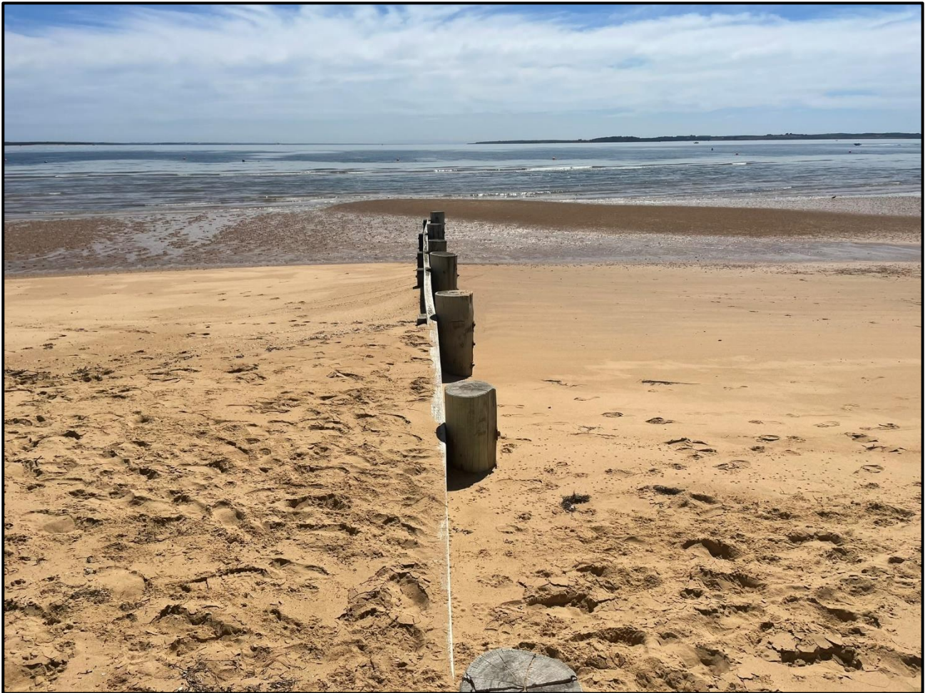
Figure 5-9: A functional groyne that retains sand to the west but allows bypassing around the tip to the east Observed on site in February 2024.
