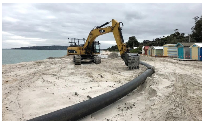
Renourishment works underway at Dromana beach, February 2021.
