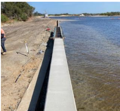
Construction of concrete capping for the Bullock Island North Arm seawall
