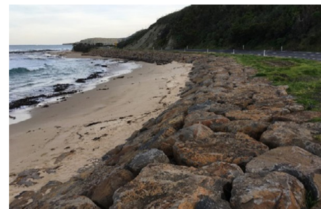
Figure 21. Rock revetment Skenes Creek
