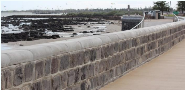
Masonry seawall at Seaholm (Photo: Alluvium)
