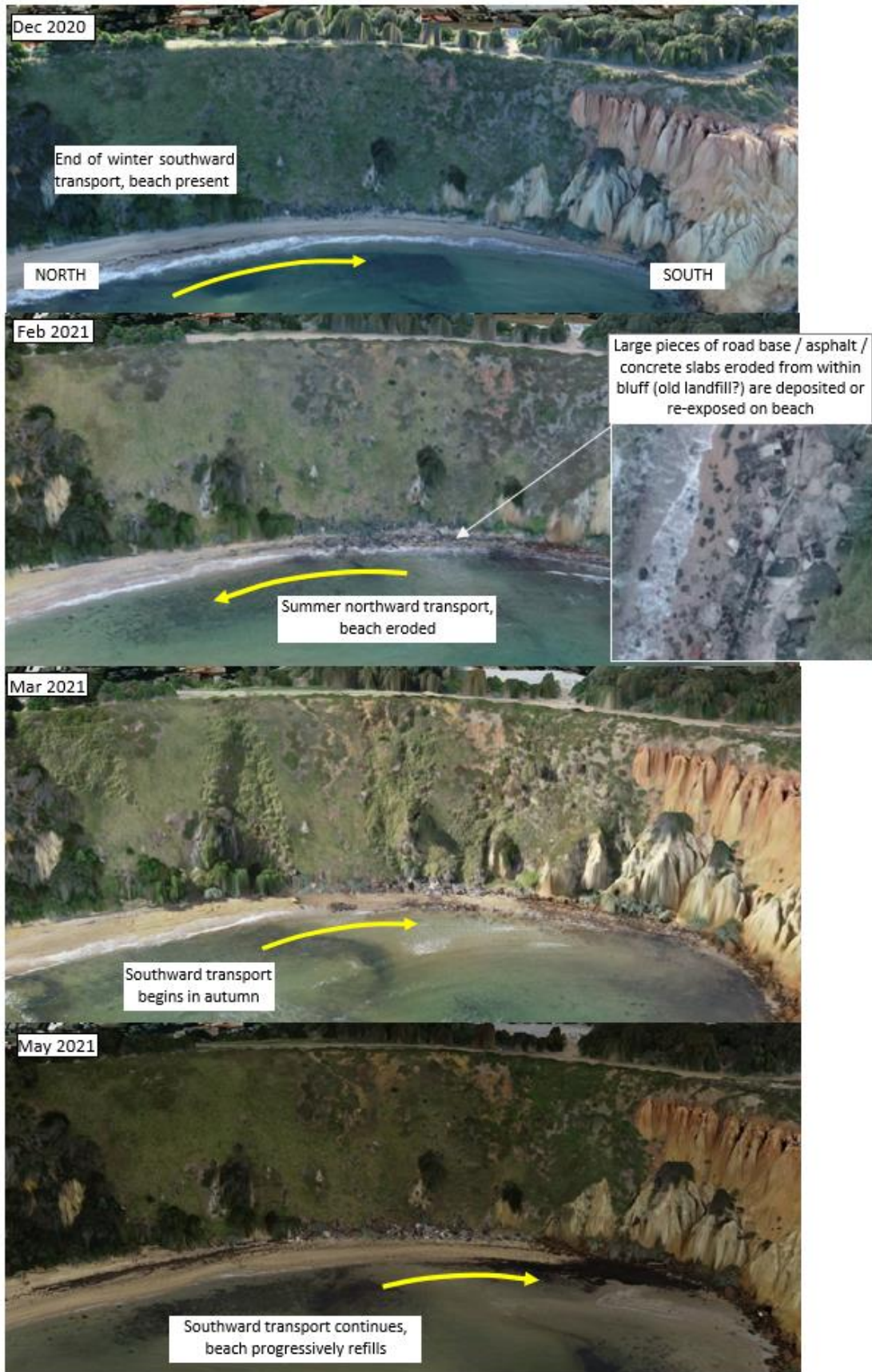
Fig. 3.3.7. Sandringham south end June 2021 nourishment site, drone 3D-orthomosaic time series. Note: The site was remediated by Bayside Council in April/May 2021 and accessible asphalt slabs were removed, some buried debris may still be present.
