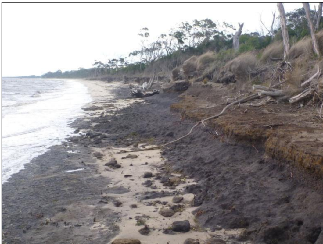
Figure 4-3 Typical Erosion of Low Earth Scarps from Western Port, Victoria
