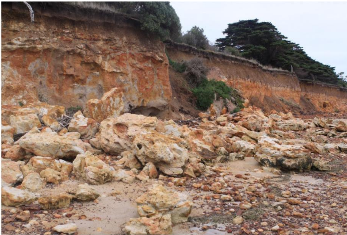
Figure 4-7 Erosion of Soft Rock Cliffs at Red Bluff (Source: N Rosengren, 2013)
