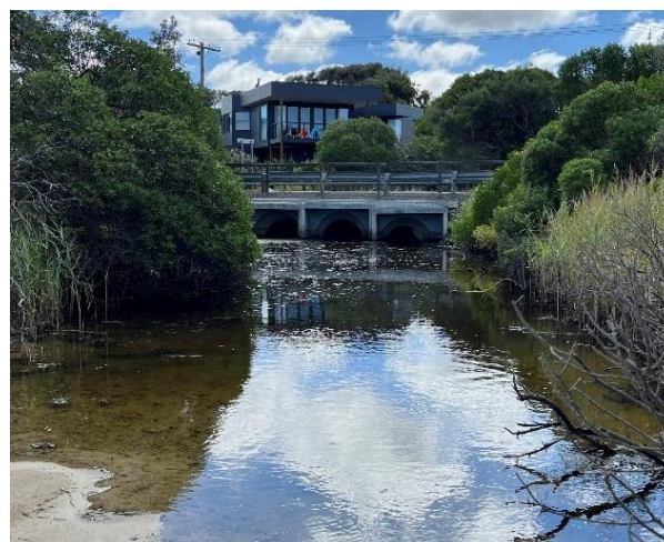
Box culverts at Wreck Creek, Inverloch. Source: Alluvium.
