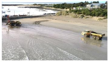
renourishment events. The renourishment works have been proposed to take sand from the beach at Wild Dog Creek (less than 1 km north-west of where the mapping ends) where it is accumulating, and from an accumulation point directly next to the harbour wall, as shown in the image (left).
