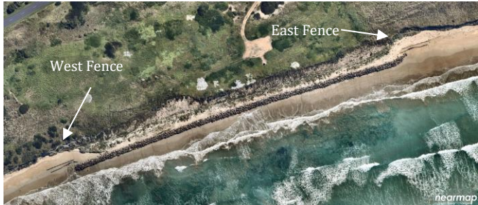
Large end scour bite behind sand fencing in the east, less pronounced end scour bite in the west. Image: Nearmap September 2021.
