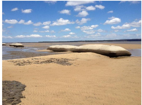
Jam Jerrup Offshore Breakwater at low tide (2013)
