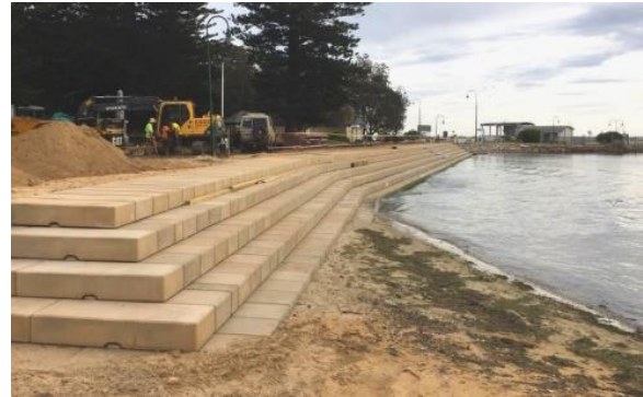
Sorrento stepped seawall
