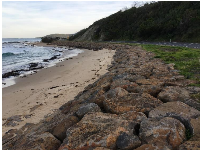
Skenes creek rock revetment adjacent to the Great Ocean Road.
