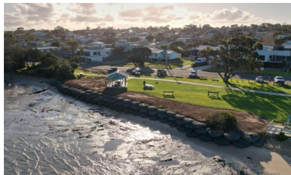
Rock Bag revetment installed at Pymble Ave reserve, Inverloch (source: engage.basscoast.vic.gov.au).
