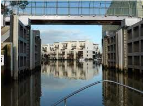
Patterson Lakes Tidal barrier – Open
