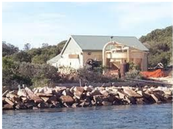
Lakes Entrance sand bypassing station (source: ssm.com.au)
