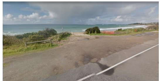
Removal of Amenities Block, Marengo, Victoria, 2010 (top), 2017 (bottom) Image source: Google street view.
