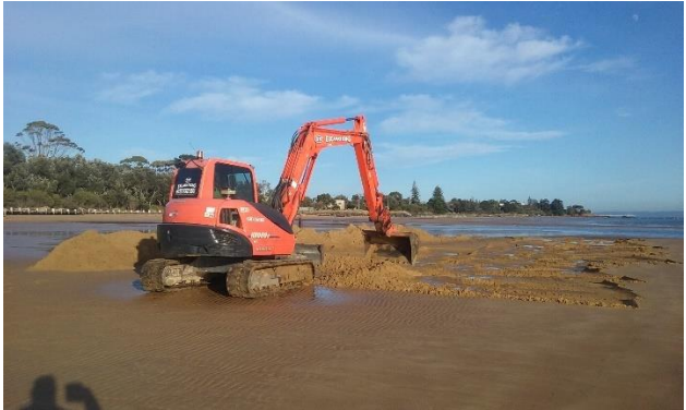
Beach scraping following a storm at Cowes East (source: Bass Coast Shire)
