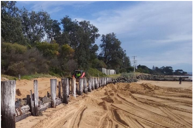
Beach scraping following a storm at Cowes East (source: Bass Coast Shire)
