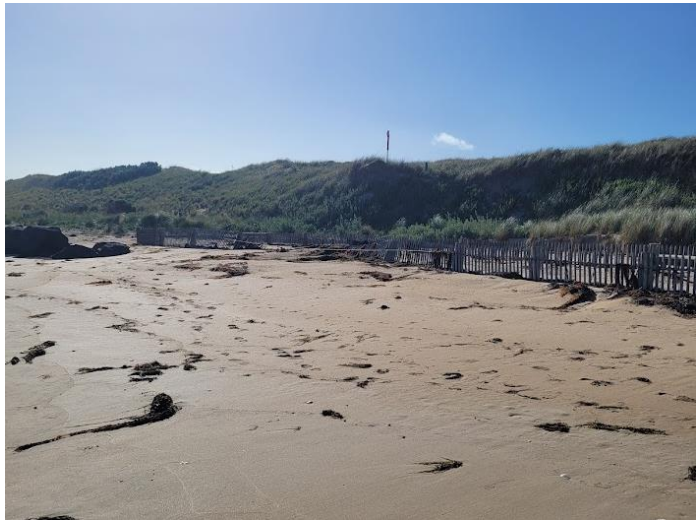
Rock structure end in the left of image and Sand fencing east of the revetment. Note the front fence has been damaged.
