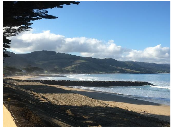
Groynes at Apollo Bay
