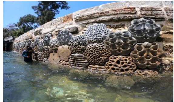
Living seawall at Sawmillers Reserve, NSW, shortly after installation (Photo by Alex Goad)
