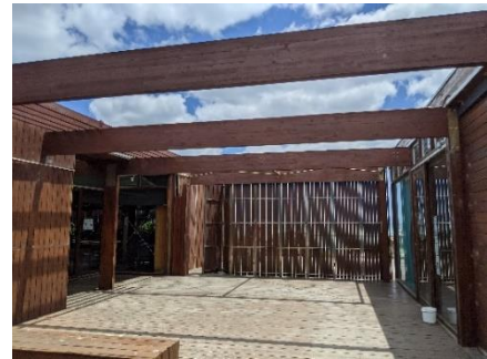
Moveable hardwood timber batten screens
