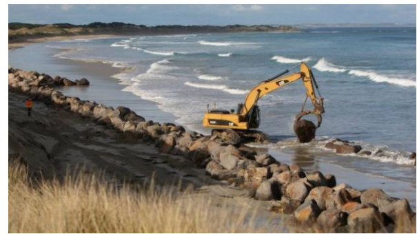
Figure 16. Construction of the wave energy dissipation structure.
