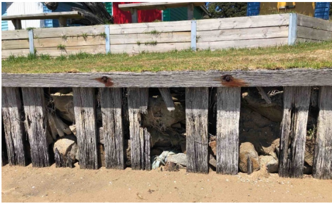
Typical missing material and decay, common in older structures.
