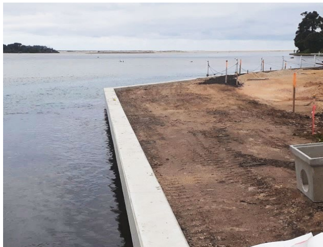
Mallacoota Foreshore seawall replacement.
