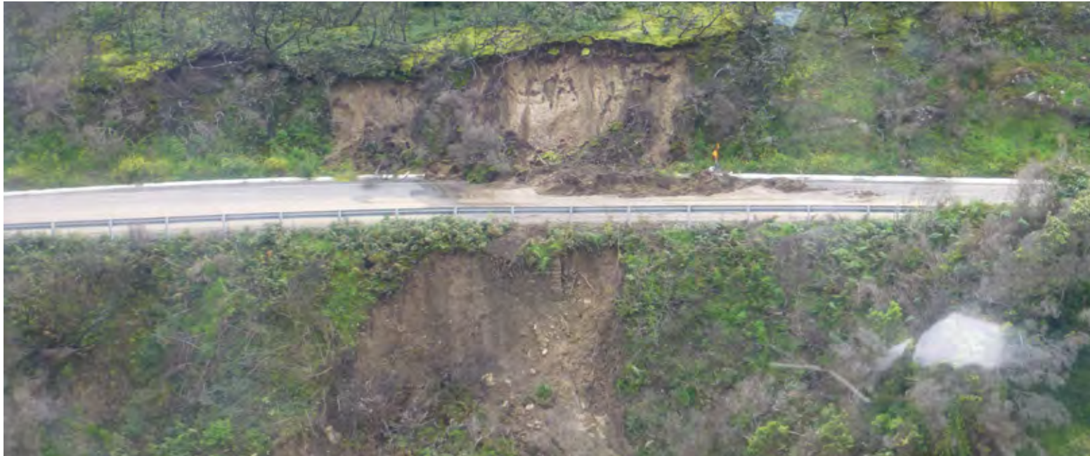
Figure 14: Landslips and erosion are a major risk along the Great Ocean Road between Lorne and Apollo Bay causing the Road to be closed periodically
