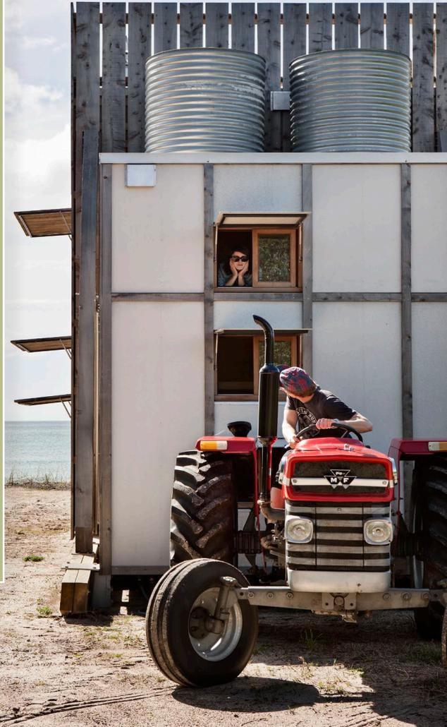
This structure incorporates innovative construction techniques to adapt to local conditions of erosion and sea level rise. The pavilion is perched on two thick wooden sleds which maximise flexibility by allowing movement around the beach as erosion or weather conditions dictate. (The Whanapoua Sled House, Coromandel Peninsula, New Zealand, Photo: Simon Devitt)
