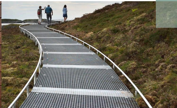
**Reinforced polymer mesh** - lightweight - chosen for its excellent anti-corrosive and low maintenance properties.
