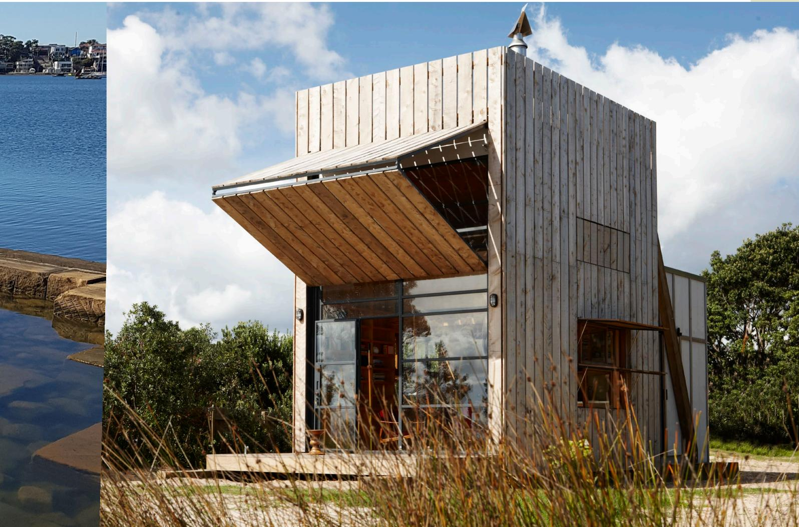
The structure is a compact building featuring sustainable water-saving waste treatment system and flexible screens. It uses ecologically friendly materials and incorporates sustainable, closed-loop systems (a worm tank system to treat waste and two tanks for grey water that can be recycled). When not in use the building is 'boarded up' and blends in amongst the dunes. (The Whanapoua Sled House, Coromandel Peninsula, New Zealand, Photo: Jackie Meiring)
