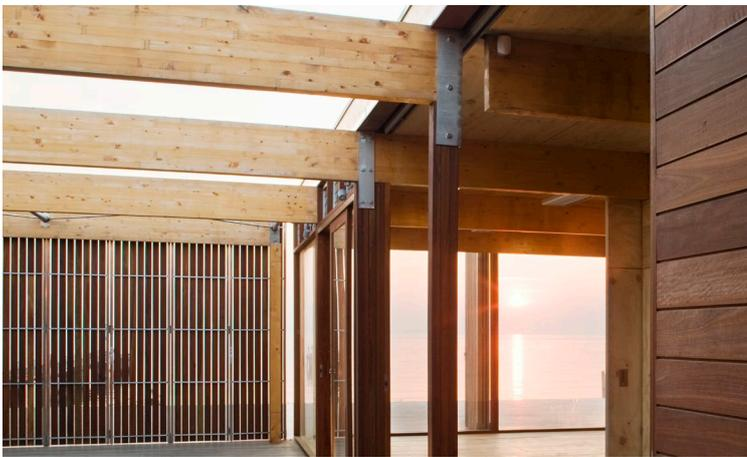
**Hardwood timber** - plantation - grown and recycled timber treated for protection from insects and decay - Red Gum, Jarrah and Tallowood are most durable and suitable for structure is the water.
