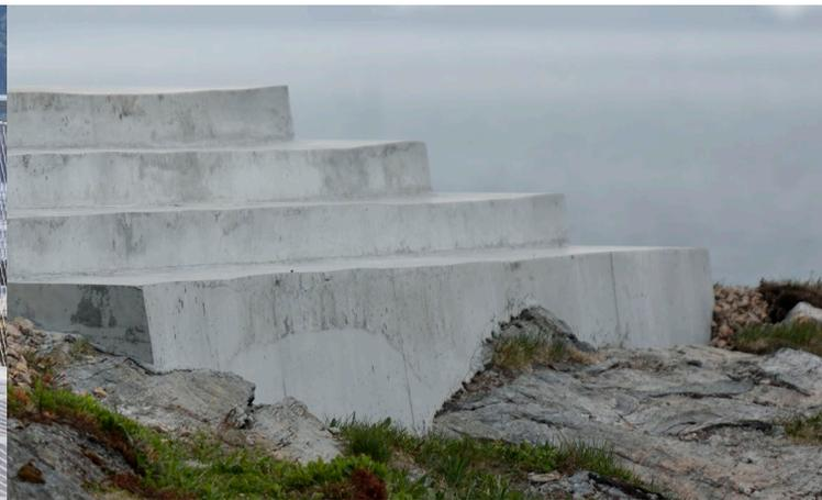
**Concrete** - durable providing there is adequate cover to all reinforcement to prevent corrosion. Photo: Jarle Waehler
