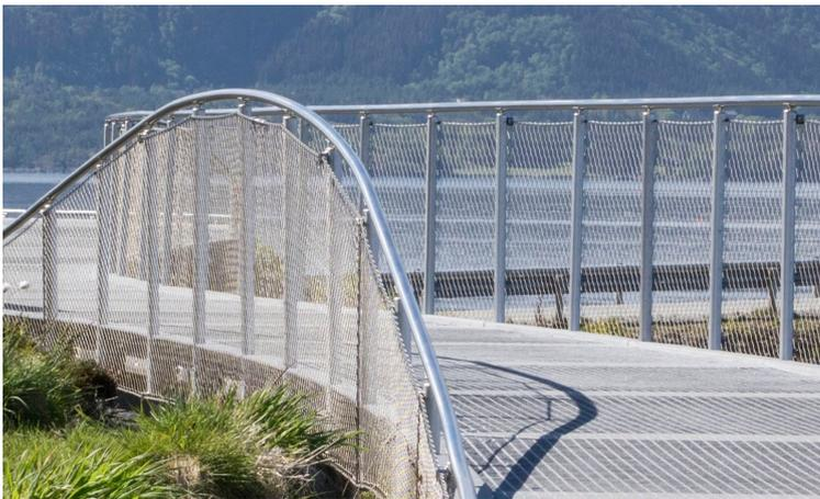
**Steel** - structural grade and hot dip galvanised as per AS/NZ 4680 for superior performance and powder coated for corrosive protection.
