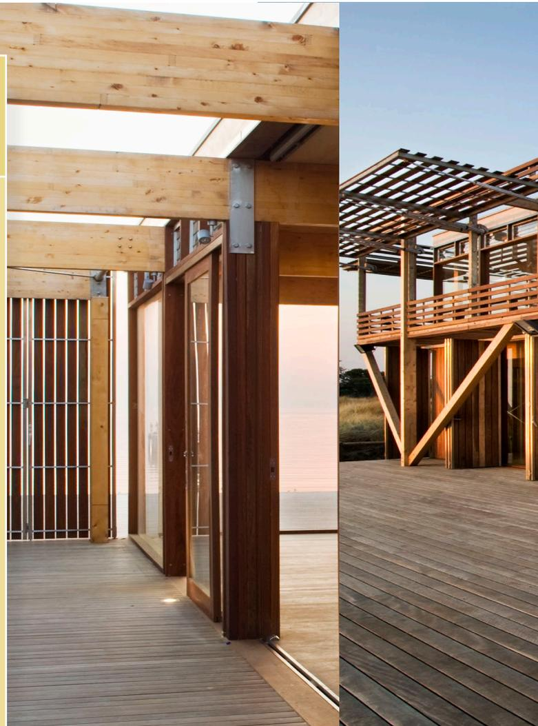
The building design optimizes thermal performance and natural light through the use of movable timber batten screens. Internal spaces can be adapted to maximise thermal comfort by moving the screens according to season and time of day. (Seaford Life Saving Club, Seaford, Design: Robert Simeoni Architects, Photo: John Gollings)
