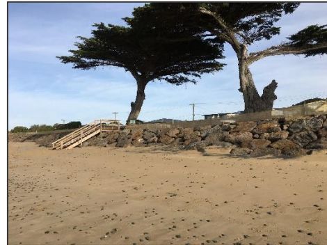
Image 2: Existing revetment at Milford St with beach access stairs.
