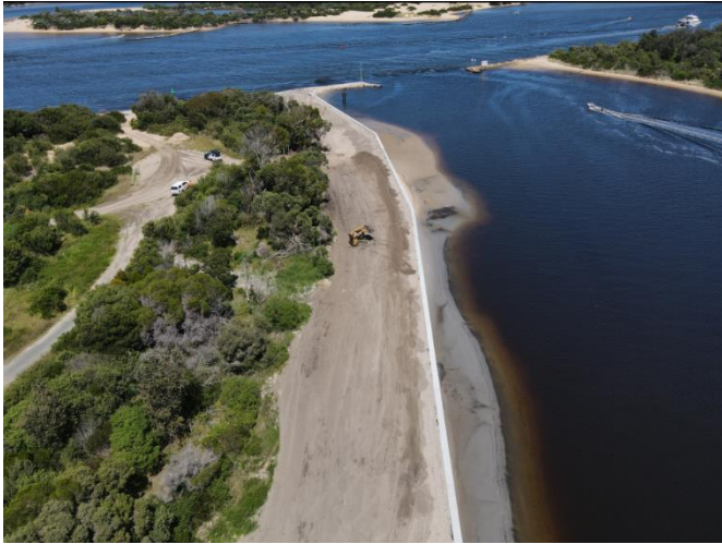
Replacement of a concrete panel seawall for the Bullock Island North Arm seawall
