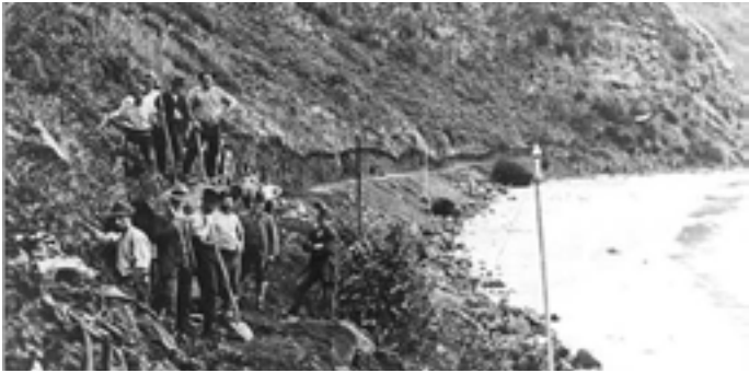
Great Ocean Road Construction workers c1920 (Source: Heritage Victoria)
