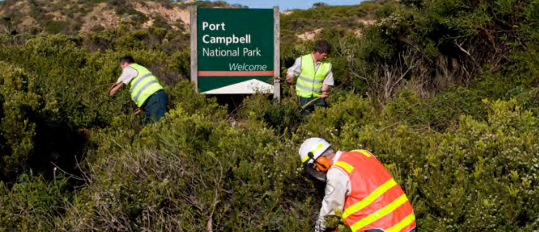
Maintenance work - Port Campbell National Park Source: Parks Victoria
