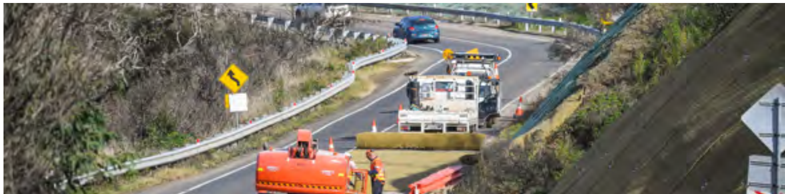
Maintenance work - Wye River Source: VicRoads
