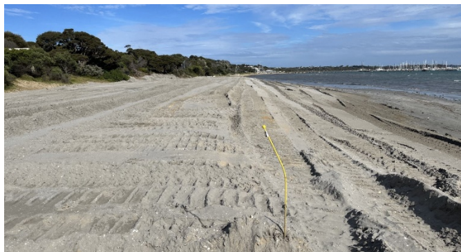
The renourished beach prior to final trimming. The sand will bleach over the coming weeks.
