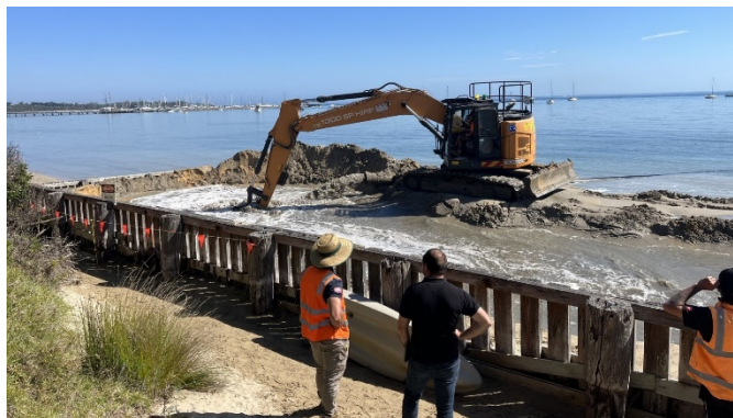
An excavator spreads the incoming sand at Blairgowrie beach.
