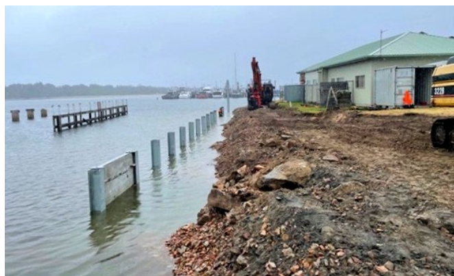
Construction of the seawall at Ocean Rescue, Lakes Entrance
