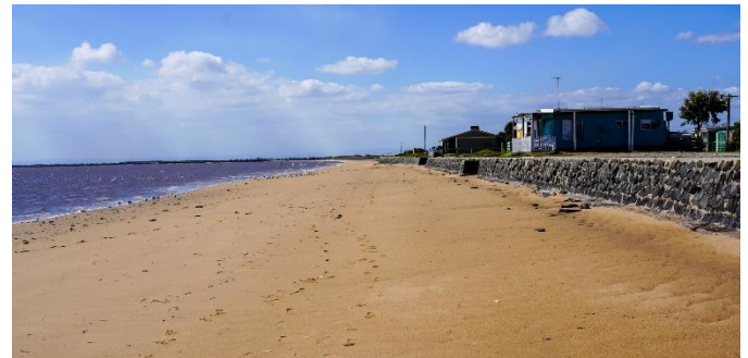
Picture 2: Seawall at Lang Lang (DEECA)
