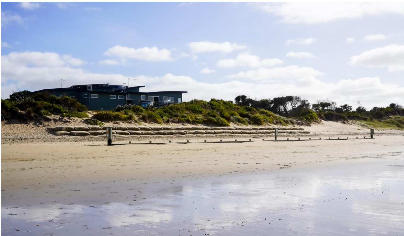
Picture 4: Sandbag seawall at Inverloch (DEECA)
