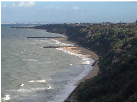
f) Looking north along Sandringham Beach, showing lee erosion on the northward side of the groyne (March 2015)
