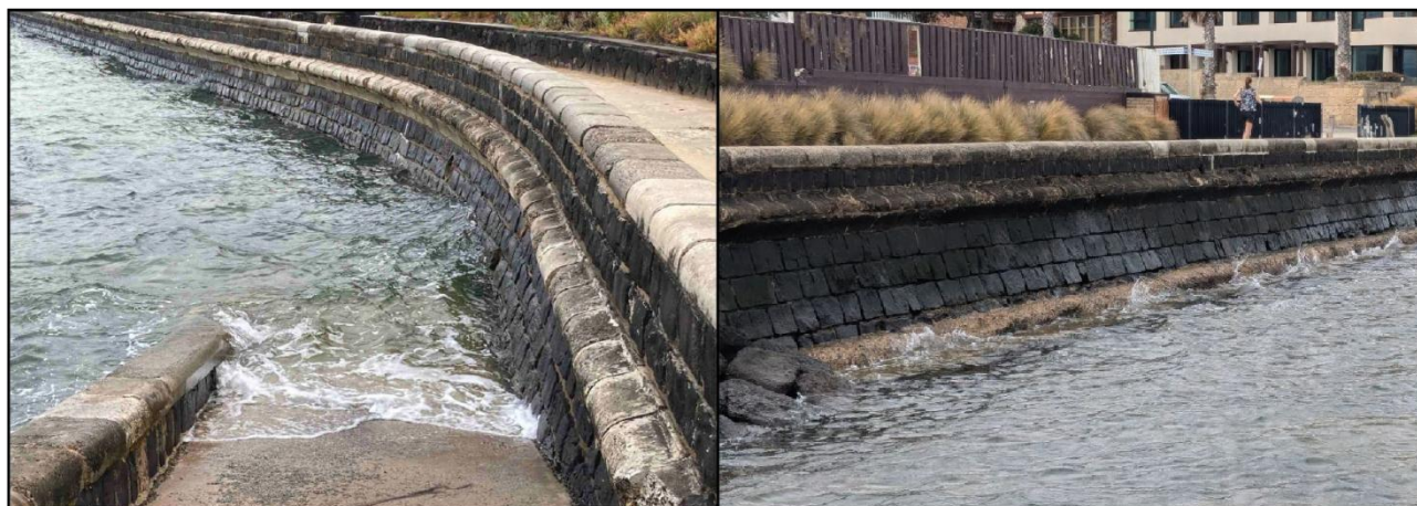
Figure 3-13: Photographs of vertical seawall
