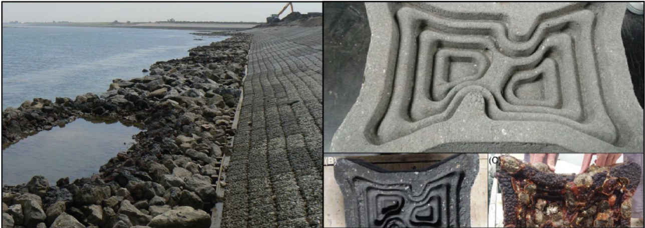
Figure 3-9: Photographs of “rich” revetment
