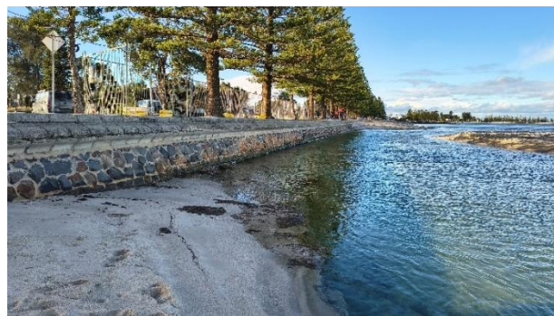
Figure 2. Flows from Laverton Creek undercutting the Altona seawall
