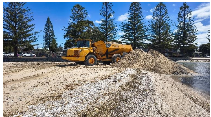
Figure 5. November 2025 construction works, including reshaping of the Altona foreshore
