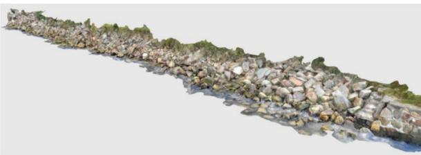
Figure 4-2 3D Scan of Seamec Rock Revetment
