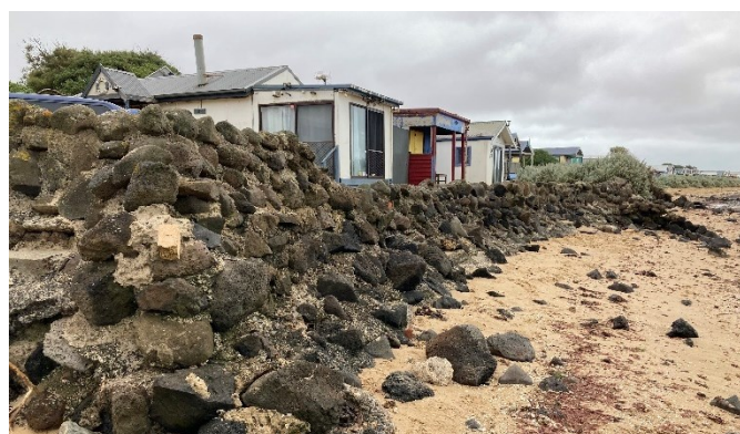
Beach erosion and degrading protection at Campbells Cove. Source: DEECA
